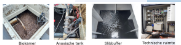
Figure 3: Overview of the different compartments in the purification container.
