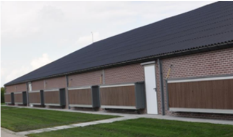
Pad cooling at the broiler house (Photo Experimental Poultry Centre)
